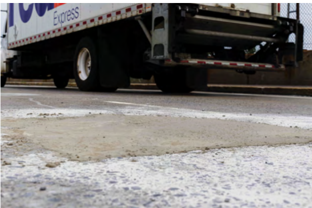
New York State DOT Bridge Deck Repairs
