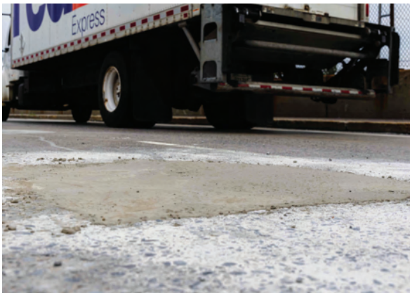
New York State DOT Bridge Deck Repairs
