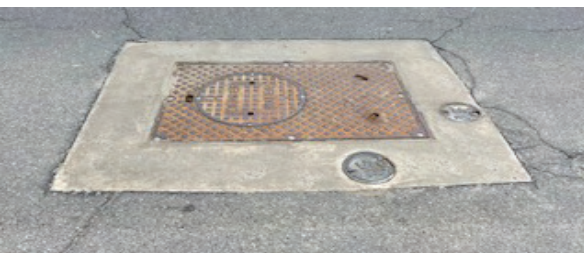
Manhole restoration to surface
