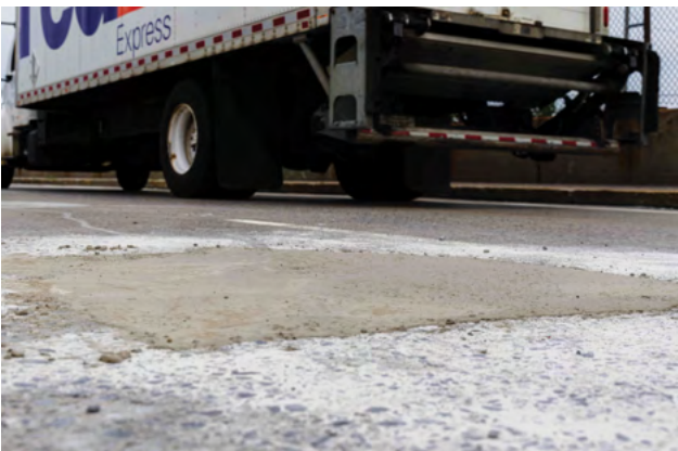
New York State DOT Bridge Deck Repairs
