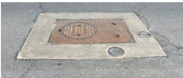
Manhole restoration to surface
