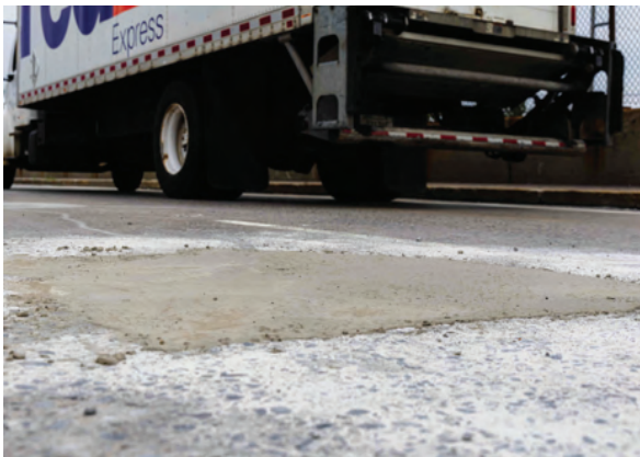
New York State DOT Bridge Deck Repairs
