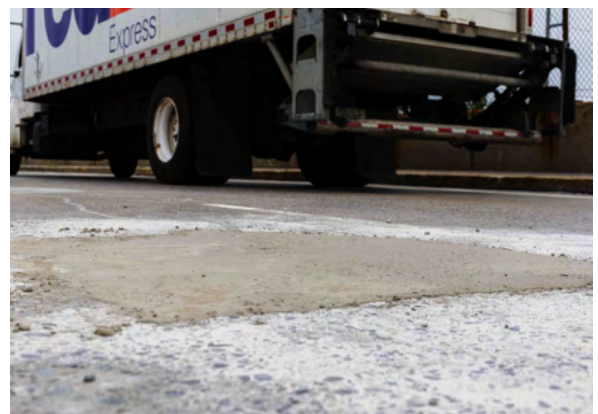
New York State DOT bridge deck repairs
