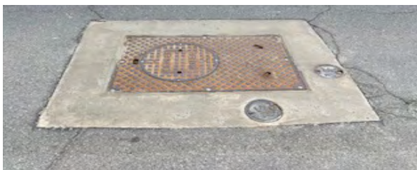
Manhole restoration to surface
