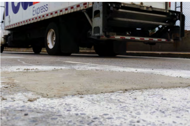
New York State DOT Bridge Deck Repairs
